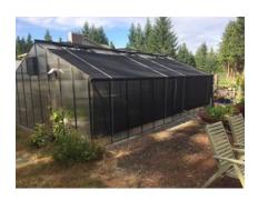
It is recommended to apply shade cloth to the outside of the greenhouse. It will absorb the excess heat without overheating the greenhouse itself. See page 2 for installation tips!
